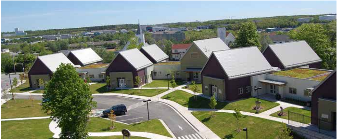
Simpson Landing, part of the Recovery and Integration service.
